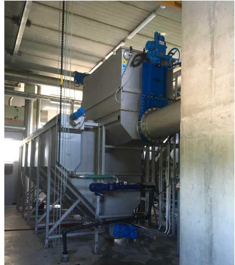
Combined screen and grit chamber
