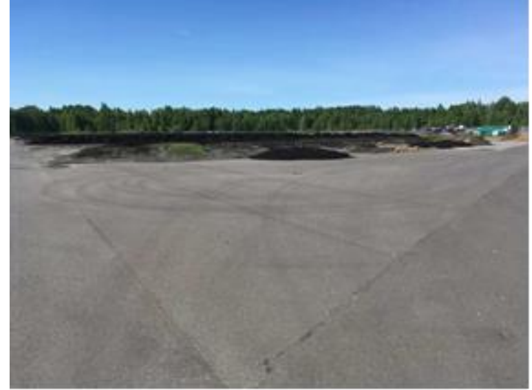
Sludge Composting plant
