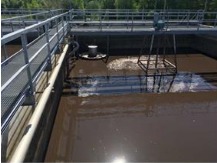
Decanter and stirrer/aerator
