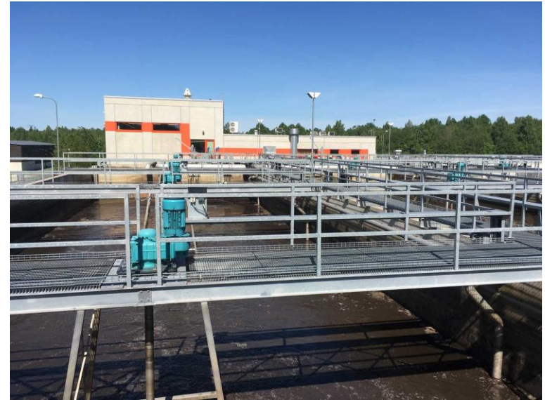
Overview Sequencing Batch Reactor
