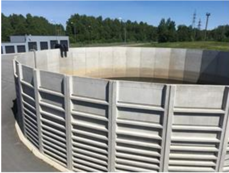
Storm water tank
