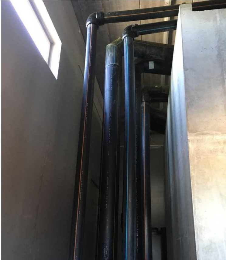
Influent pressure pipes
